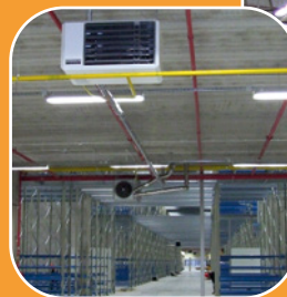
Project in Ireland by JF McKenna. New poultry house with 50.000 chickens with 4 DXE heaters.
